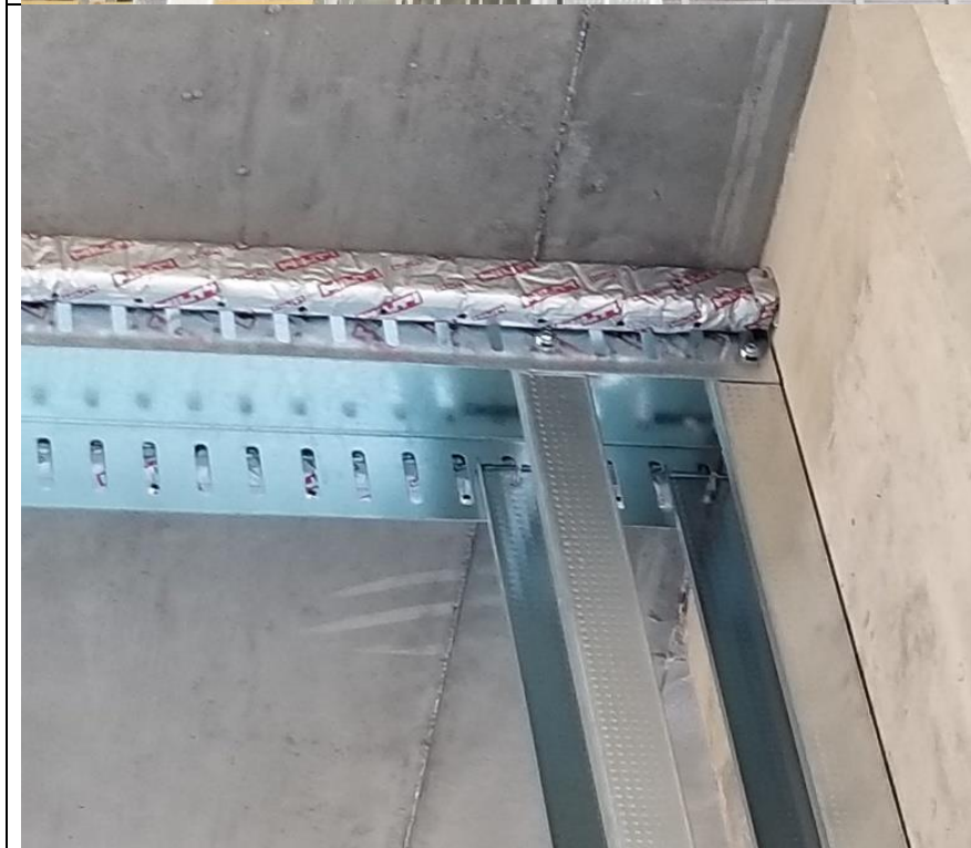
Top of wall framing showing Hilti CFS-TTS installation
