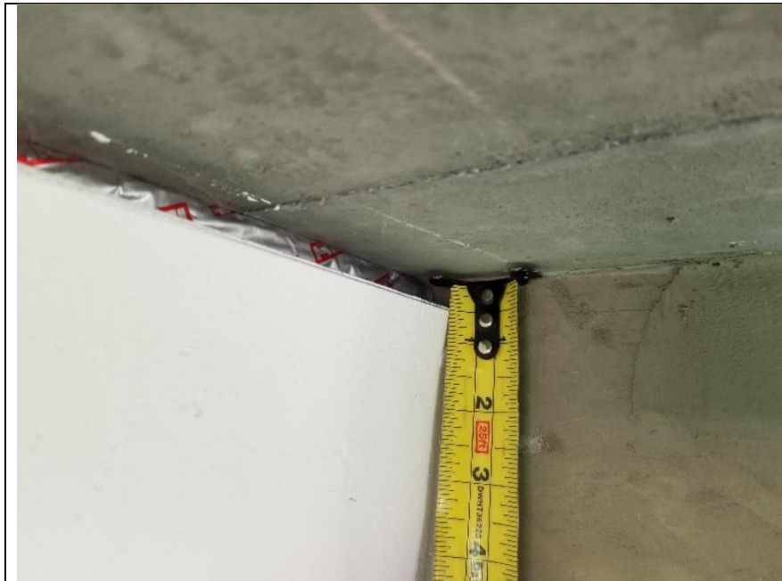
Top of wall showing Hilti CFS-TTS and 1/2-inch clear
