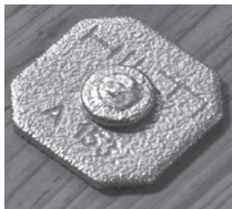
Installed X-CP fastener with "A 153" clearly marked on washer.
