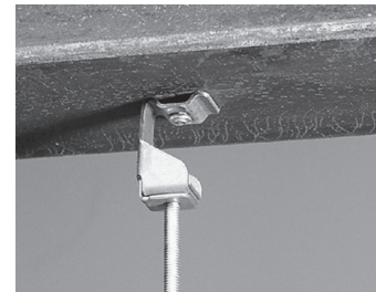
Threaded and smooth rod hangers
