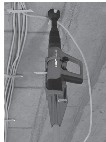
Cable and conduit attachment
