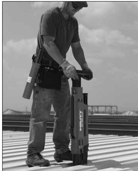
Fastening with the DX 860-ENP-L
