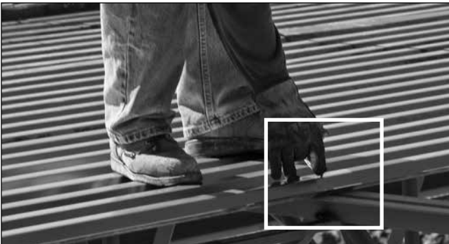
Fastening with the DX 860-ENP-L
