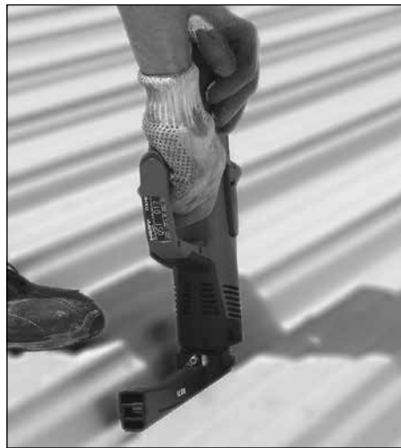
Fastening with the DX 76-MX
