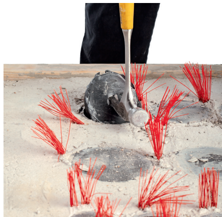
Figure 15 — The Hilti CFS-CIS MD fire stop system for composite floor decks
