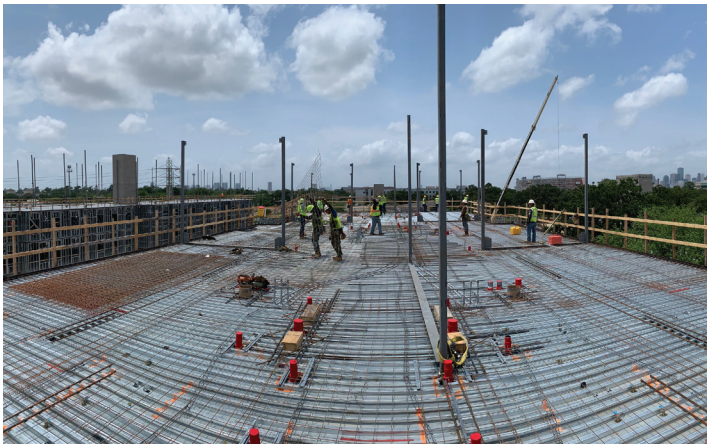
Figure 1 — Composite floor deck construction
