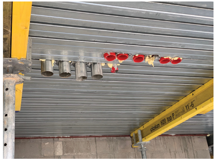
Figure 12 — An example of through-penetration firestop system
