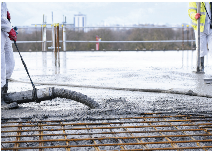
Figure 5 — Construction of composite floor deck
