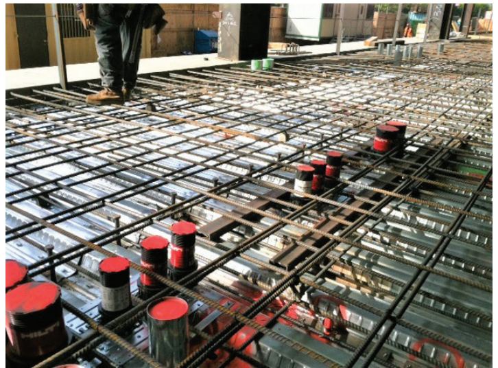
Figure 2 — Penetrations in composite floor decks
