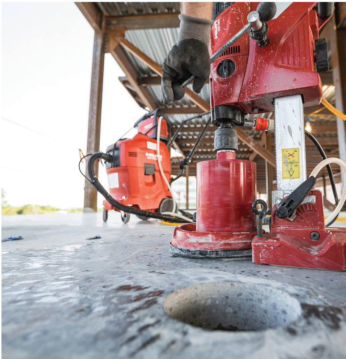
Figure 13 — An example of core-drilling of a concrete floor
