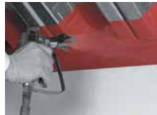
Superior finish smooth surface allows quick and cost effective coverage with Hilti CFS-SP WB Firestop Joint Spray.
